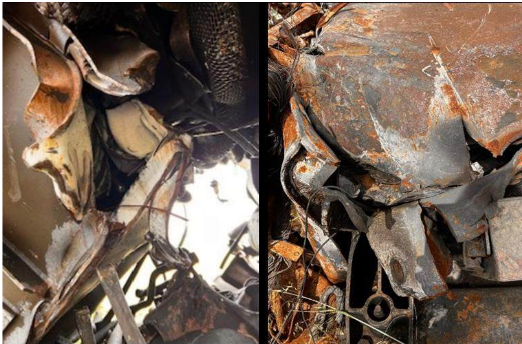
Figure 67. Large cracks of the transformer still attached under the 120-022 locomotive (Left). Bumps, folds, rips and large cracks of remaining locomotive transformer 120-023 (right), see also Figure 61.
