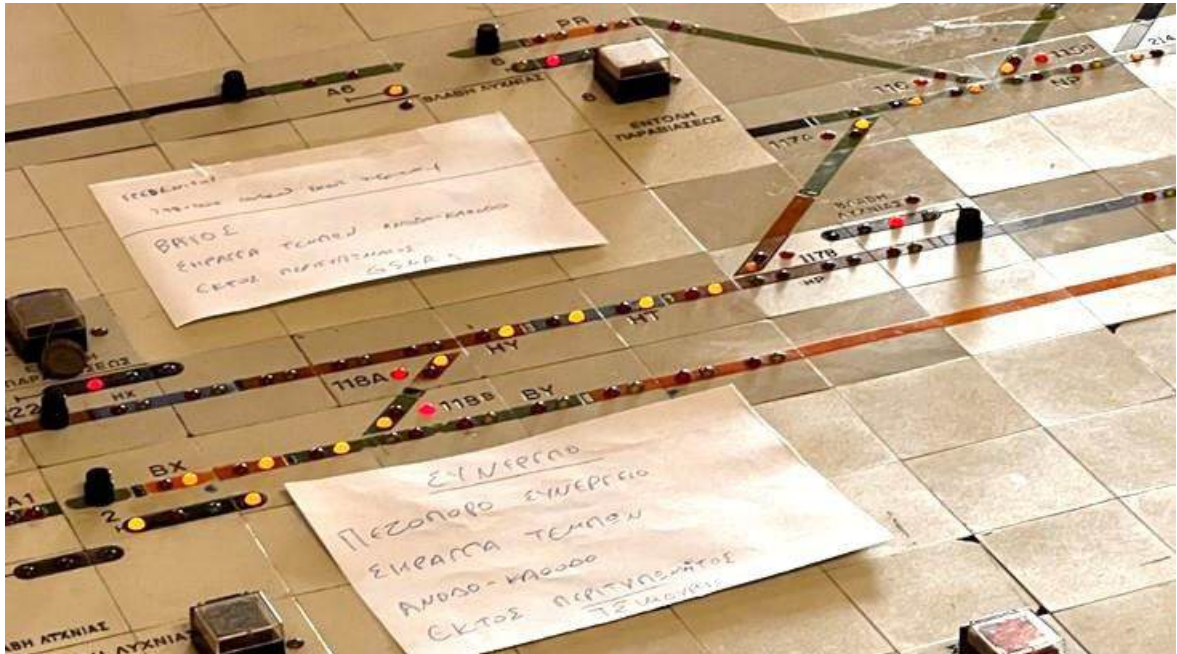
Figure 48. Detail of the Larissa Control Panel with a route set to cross a switch in a bypass position.
