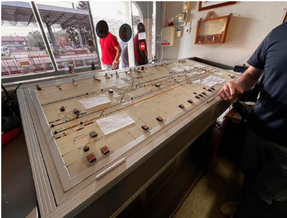
Figure 37. The control panel at Larissa Station
